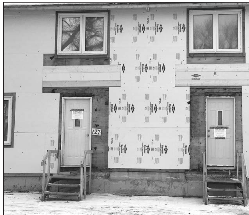
Homes on the Base which are under renovations often see asbestos removed (left) before work commences on both interior and exterior (right). Besides new windows, doors and siding, work is done on new front or side entrance steps.
