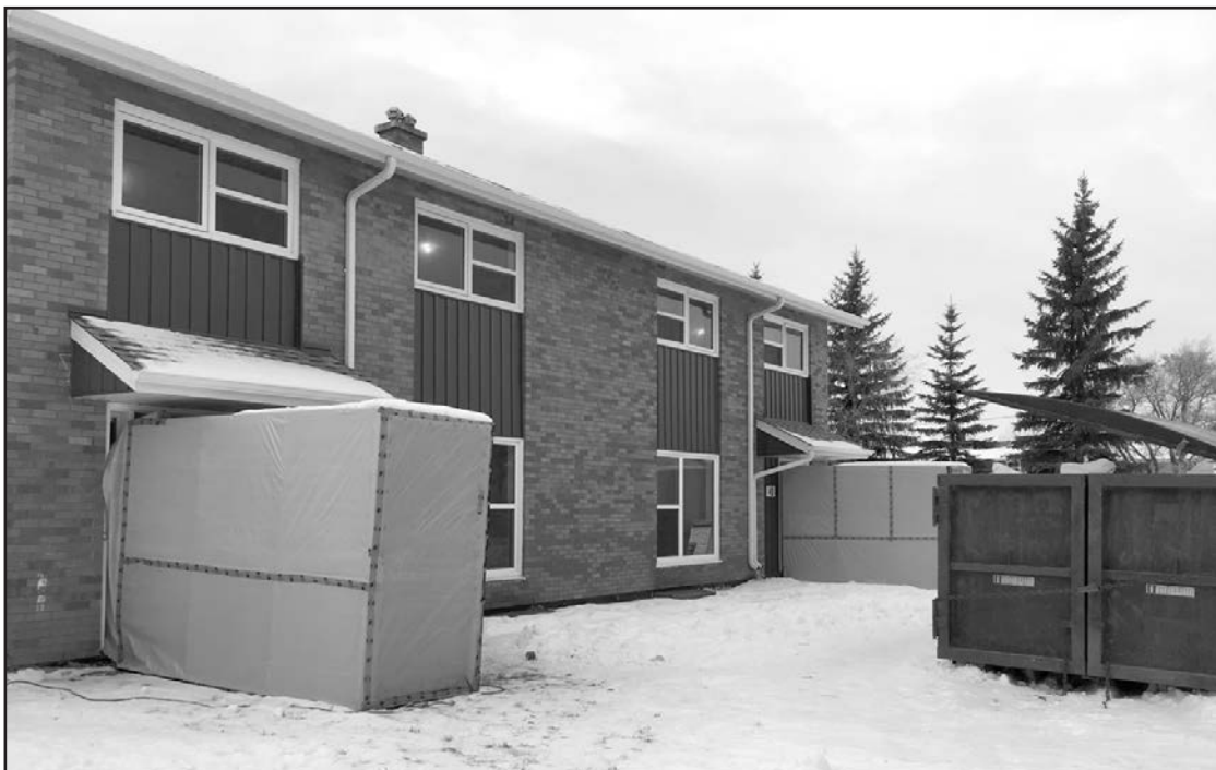
Homes on the Base which are under renovations often see asbestos removed (left) before work commences on both interior and exterior (right). Besides new windows, doors and siding, work is done on new front or side entrance steps.
