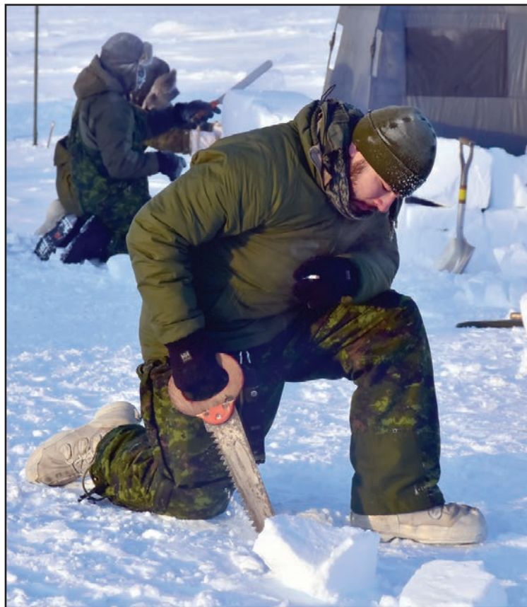
A special saw is used to carve out snow blocks used by 2PPCLI to build snow walls around their tents to keep the Arctic chill away from their sleeping quarters.
