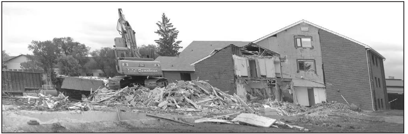
The Leslie Barracks was demolished last summer.
