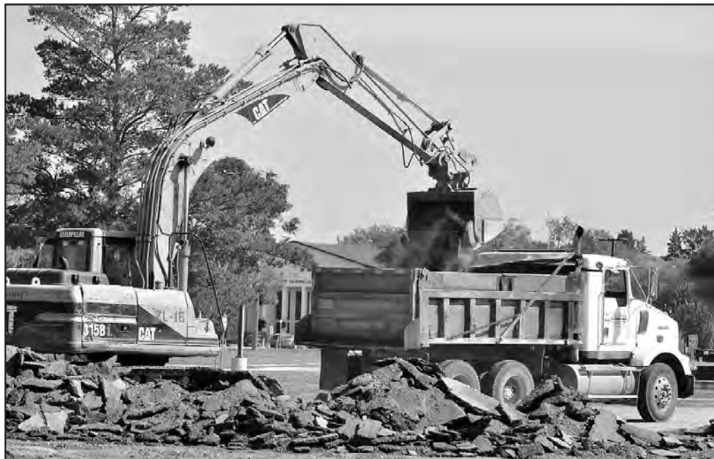
Preparing for the new asphalt on the parking lot west of the GSH, work crews have been busy removing the old pavement (left). Additional earth was removed next, then fresh earth brought in and leveled. PMQs 40, 38, 36 and 34 are no more (right) after a demolition crew from Cumming and Dobbie took the defunct homes down on Kingston Avenue. There are five more similar duplexes to be removed once the asbestos is removed.
