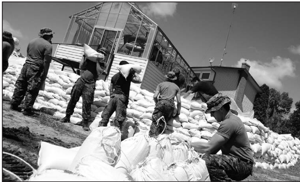
Sandbags placed around a home in the flood zone by IRU troops.
