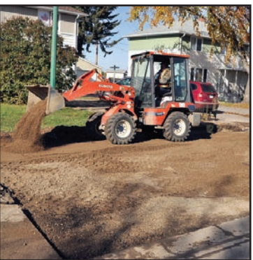
Kingston Avenue paving repairs underway. Page 8
