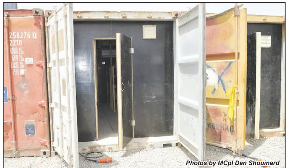
Above, members of the MTTF Engineer Squadron install interior walls in a sea container they are converting into a barrack room for Afghan soldiers. When finished, each accommodation seacan as seen below has bedspaces for up to 10 soldiers, with lighting, electric outlets, an air conditioner, and a base plate to support a wood stove for cooking and space heating.
