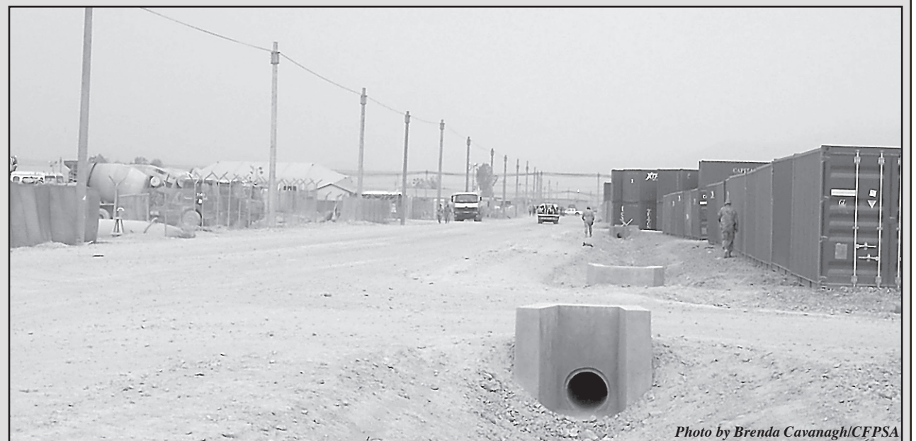
Main street at the Kandahar Airfield Field in Afghanistan.
