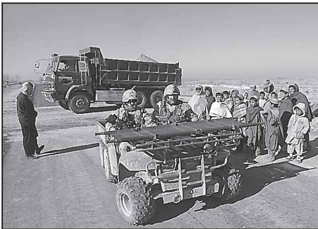
As roadwork continues nearby, Engineers overseeing the project inspect sections of Route Summit that have already been completed. The road, completed by local workers and contractors will connect the busy District Center of Bazari Panjwayi to Highway 1.
