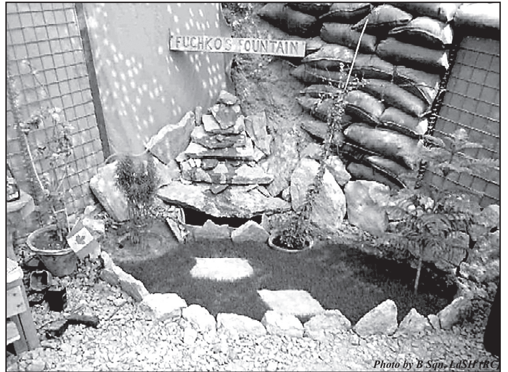
The completed "Fuchko's Fountain" project in B Sqn's expanded common area behind the troops' shacks at a Panjwayi FOB.
